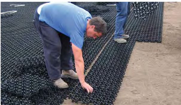
TurfPave® XD modules securely interlock and conform to uneven surfaces
