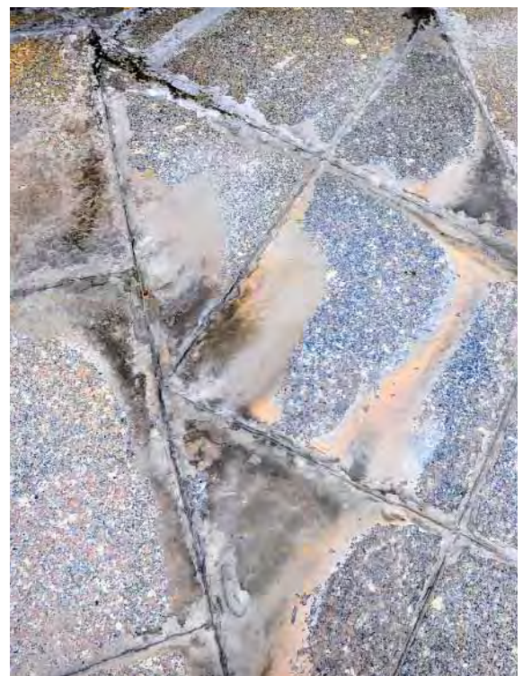
Unsightly efflorescence
